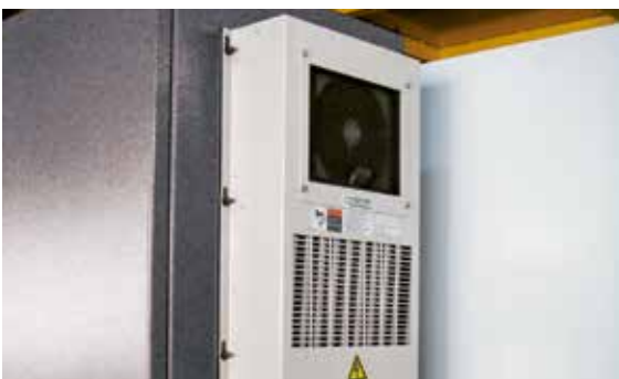
Heat Exchanger For Electrical Cabinet
